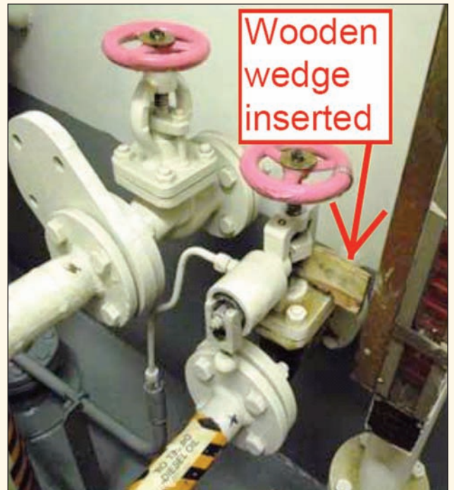
▲ QCV disabled by inserting a wooden wedge
