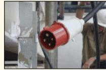
▲ Unsafe live male plug with exposed conductors
