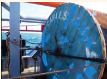
▲ View of unpacked wooden cable reel – note very narrow central hole with lifting wire sling rove through, chain and tugger wire tightened at mid-height.
