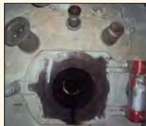
▲ View of burner assembly port showing evidence of oil accumulation
