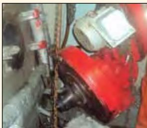
▲ Burner assembly removed and atomizer holes found blocked by unburnt residue and debris
