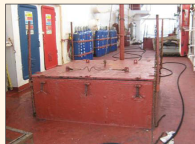
◀ View of hatchway showing portable lid and base of lifting davit
