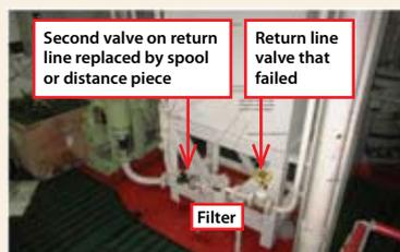
Corrective action completed – redundant valve replaced by spacer pipe
