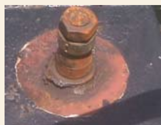
View of failed fairlead roller showing the spindle and sheared base
