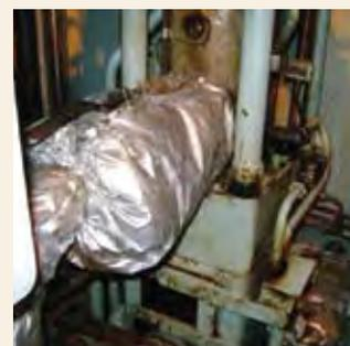
Corrective action implemented – fuel inlet pipe re-connected with new gasket and covered with insulation and containment covering
