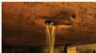
Hole in way of fore peak tank after bollard was removed
