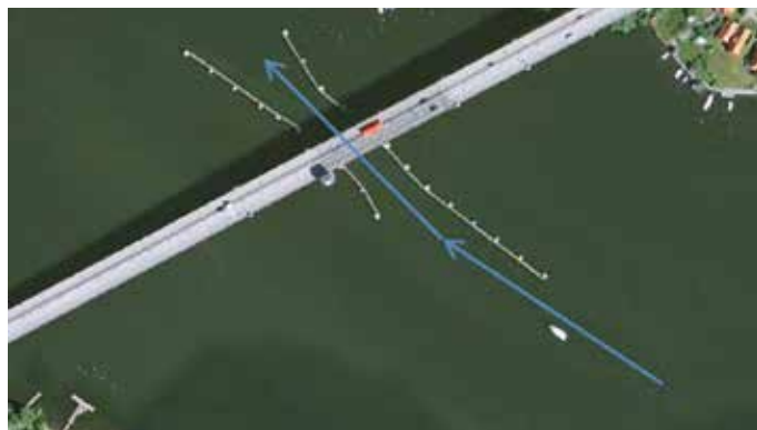
Normal approach to bridge (fendering can be seen on either side)
