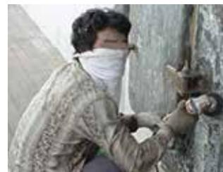
Operators of grinding and cutting tools should assume that the disc may shatter and should ensure that the guarding will deflect broken pieces away from themselves. The correct component parts which support and secure discs must always be used.
