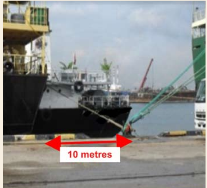
Unsafe overhang severely restricts manoeuvring room for the vessel berthed astern and increases risk of contact during mooring/unmooring
