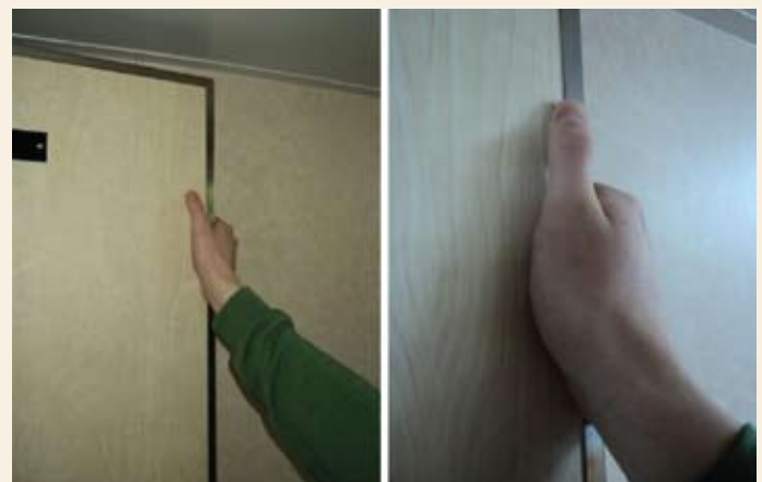
Peripheral strip edges can be as sharp as a knife blade. Crewmembers engaged in any type of work on the doors and fittings must take all precautions and don appropriate PPE.
