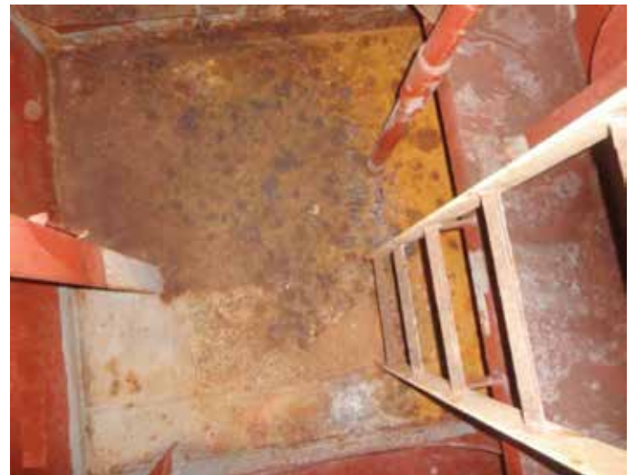
View of part of the hold access ladder
