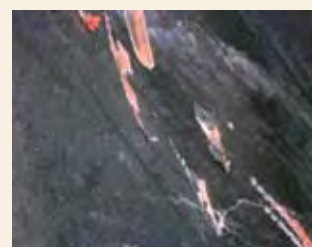
Deep gouges on topsides of own ship caused by deflated fender's metal fittings
